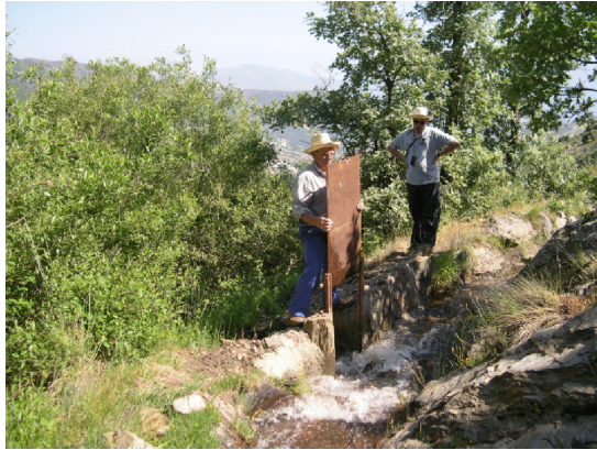
Figure 3 Acequero operating a turnout, Acequia Nueva, Poqueira watershed, Spain
