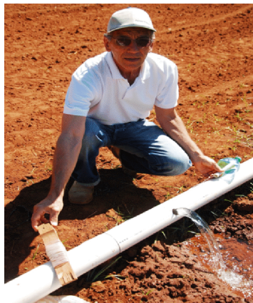
Figure 8 Fishing rope and PET bottle to retain the flow in the sewage pipe
