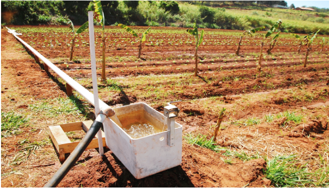
Figure 9 Small receiving box and the fishing rope attached to an adapted wire stretcher to displace the PET bottle inside the pipe
